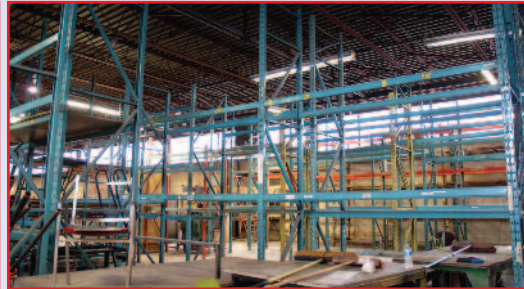
Partial View Of Pallet Racking
