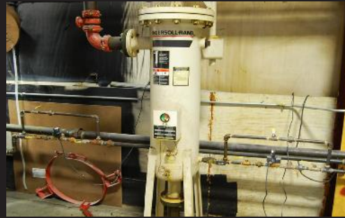
Ingersoll Rand TR1500CHE compressed air filter, 1500 scfm, 200 psig
