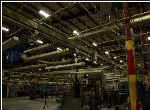
Square D bus bar and plugs; hundreds of feet
