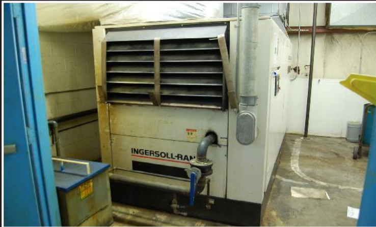
Ingersoll Rand SSR EPE 200 2S rotary air compressor; 200 hp, 125 psig rated operating pressure, 990 cfm capacity, 78,870 total hours & 60238 load hours, serial FF1951V00169
