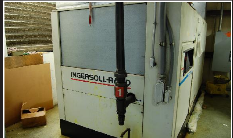
Ingersoll Rand SSR-EP150 rotary air compressor; 150 hp, 1245 psig rated operating pressure, 670 cfm capacity, 59,781 total hours, 37,052 load hours, serial F13326U96157
