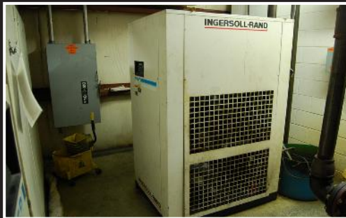
Ingersoll Rand DXR750A compressed air dryer; 1996 vintage, serial 96BDXR0794
