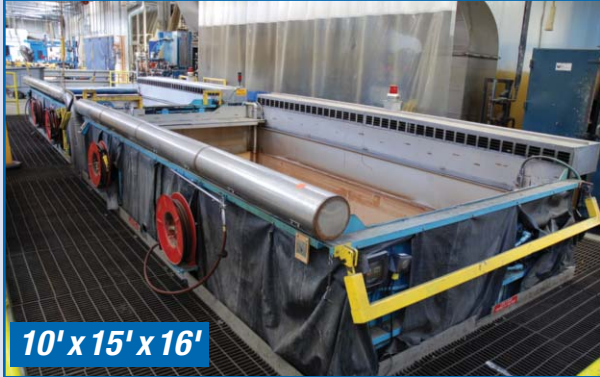
(2) METCHEM AQUEOUS WASH SYSTEM TANKS
