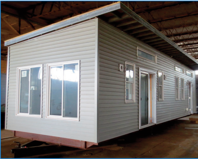
40FT X 14FT TRAILER WITH UNFINISHED EXTERIOR AND INTERIOR
