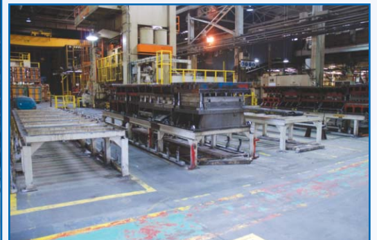
PARTIAL VIEW OF CLAMP SETS
