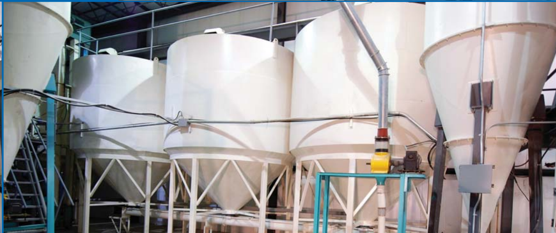
PARTIAL VIEW OF STORAGE SILOS
