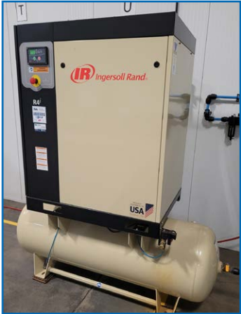
INGERSOLL RAND R4I-A145 COMPRESSOR DONALDSON TORIT DUST COLLECTOR
