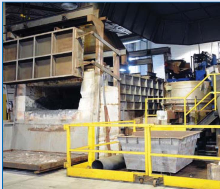
CANENG NATURAL GAS FIRED REVERBERATORY MELTING FURNACE
